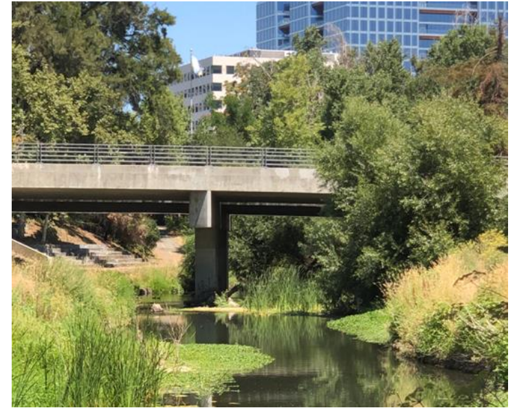
Bridge along Guadalupe River
