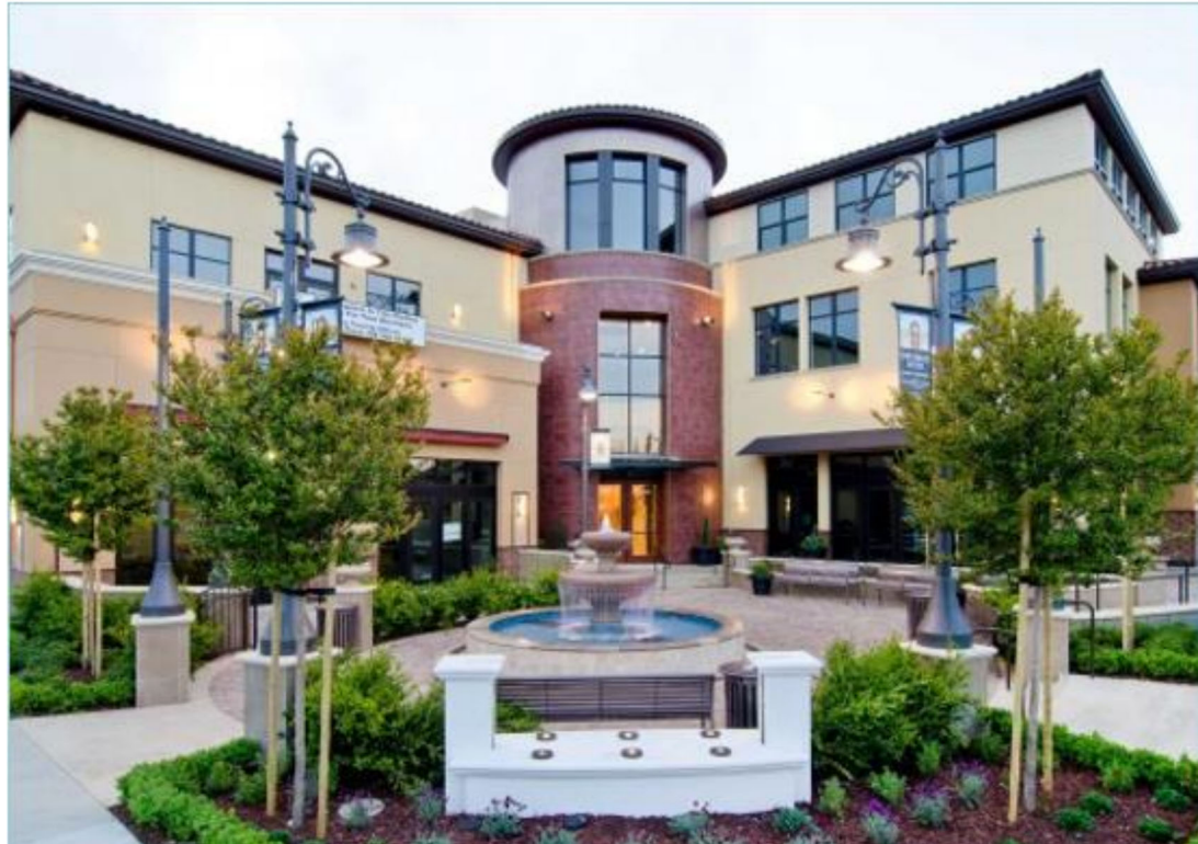
View of a publicly accessible plaza on the southeast corner of Lincoln Avenue and Willow Street – San Jose, CA https://www.wlbutler.com/project/willow-glen-town-square/
