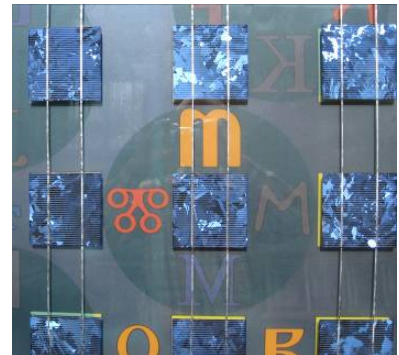
Windows – interior view (right); exterior detail of photovoltaic cells (below)
