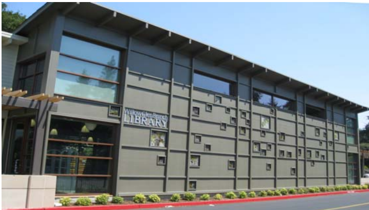
A portion of the Library's west wall, with some of the artist's windows
