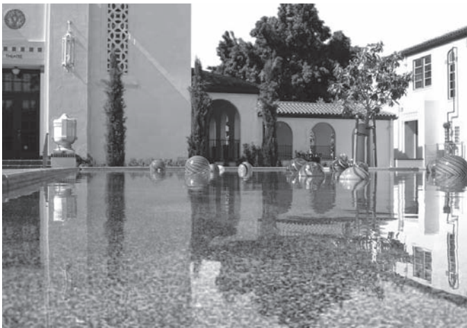
Campbell Community Center
