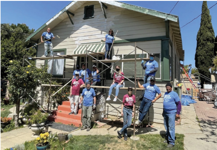
Photo via Rebuilding Together Silicon Valley
